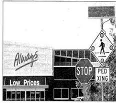
PROTOTYPE: This Texas Wal-Mart uses such green technology as solar-powered crossing signs and radiant floor heating.
